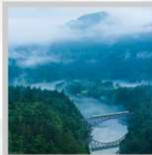
"TADAMI FIRST BRIDGE"
