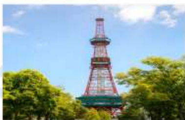
SAPPORO TV TOWER // CLOCK TOWER (VIA)
